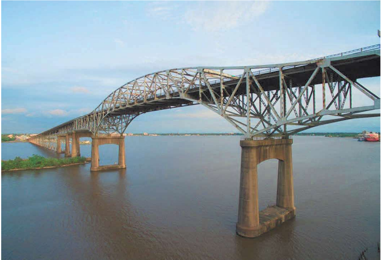
Figure 1 – I-10 Calcasieu River Bridge
