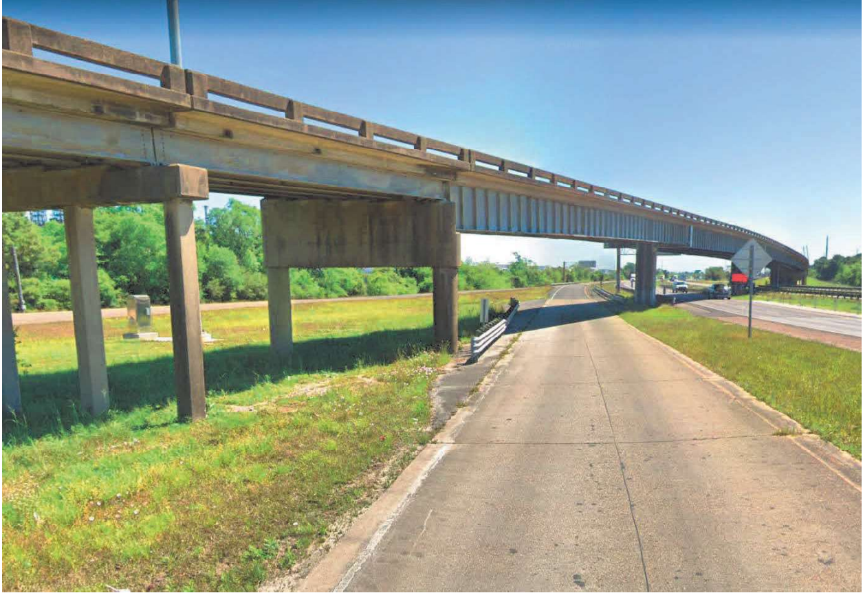
Figure 1 – US 90 Bridge over I-10
